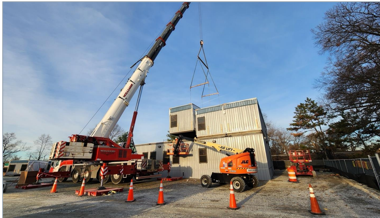
Field office construction in NPS Ball Field
