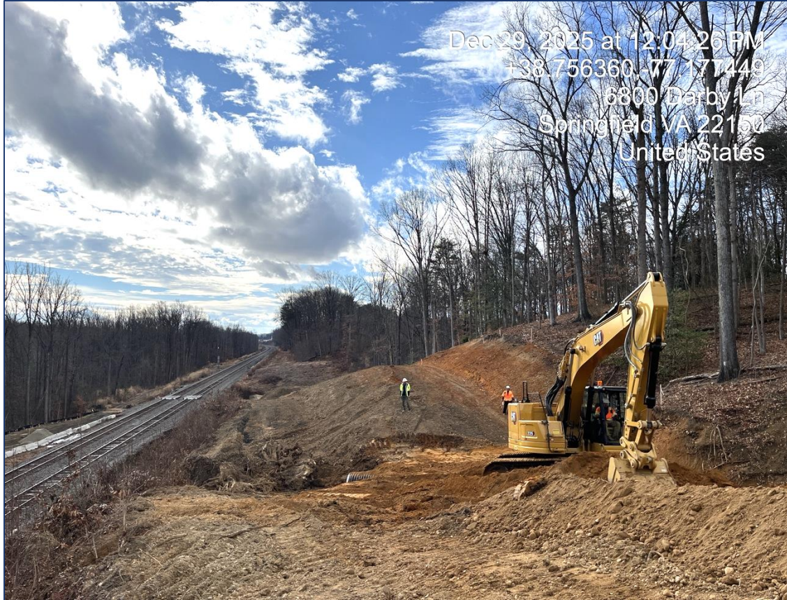
Excavation and grading for retaining wall construction
