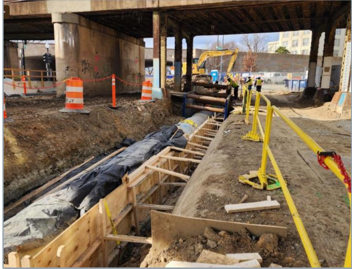
Storm sewer relocation
