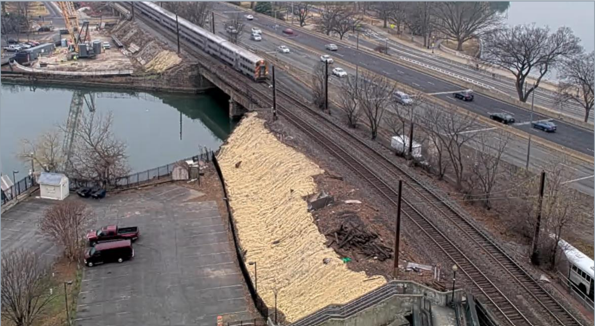
Selective Tree Clearing completed in early November
