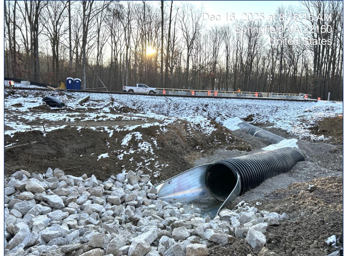
Temporary drainage installation
