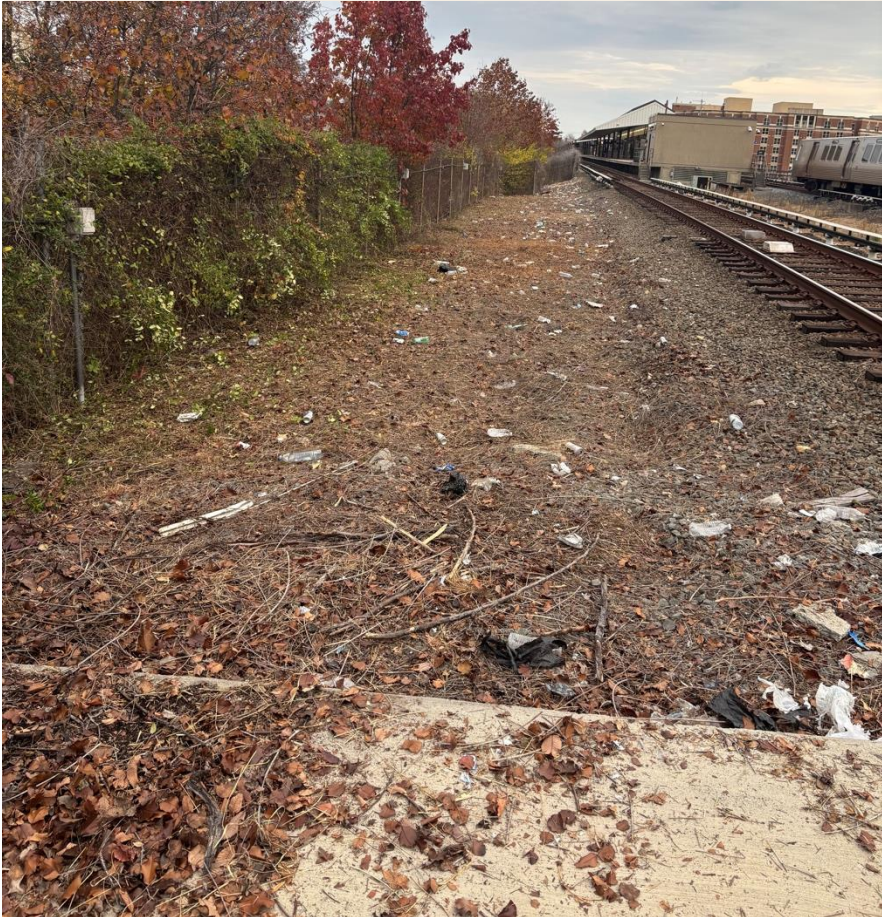
Brush clearing ahead of WMATA fence relocation
