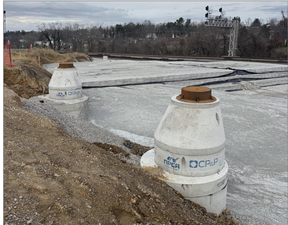
Storm sewer installation
