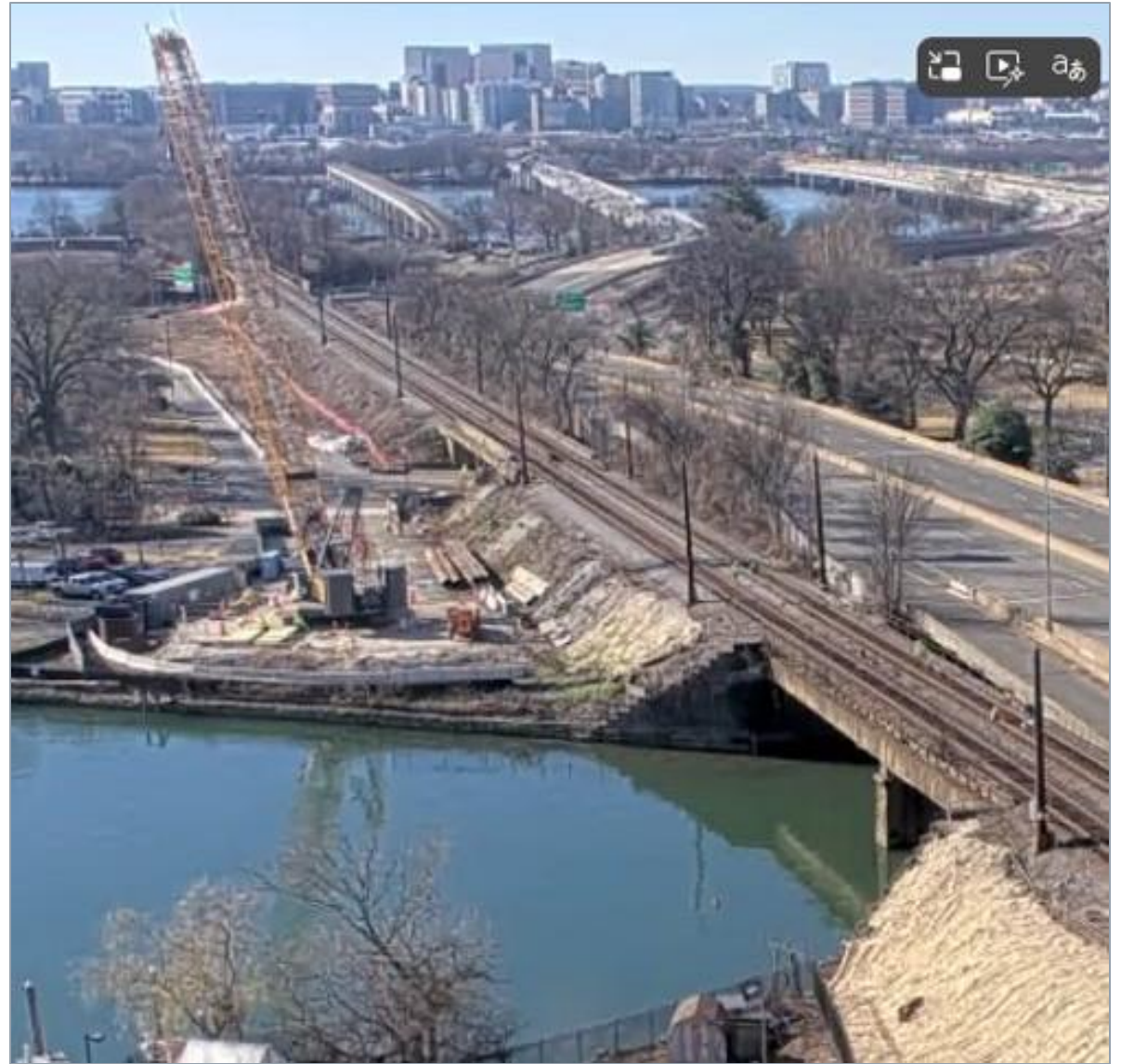
Preparing to begin construction of Washington Channel Trestle
