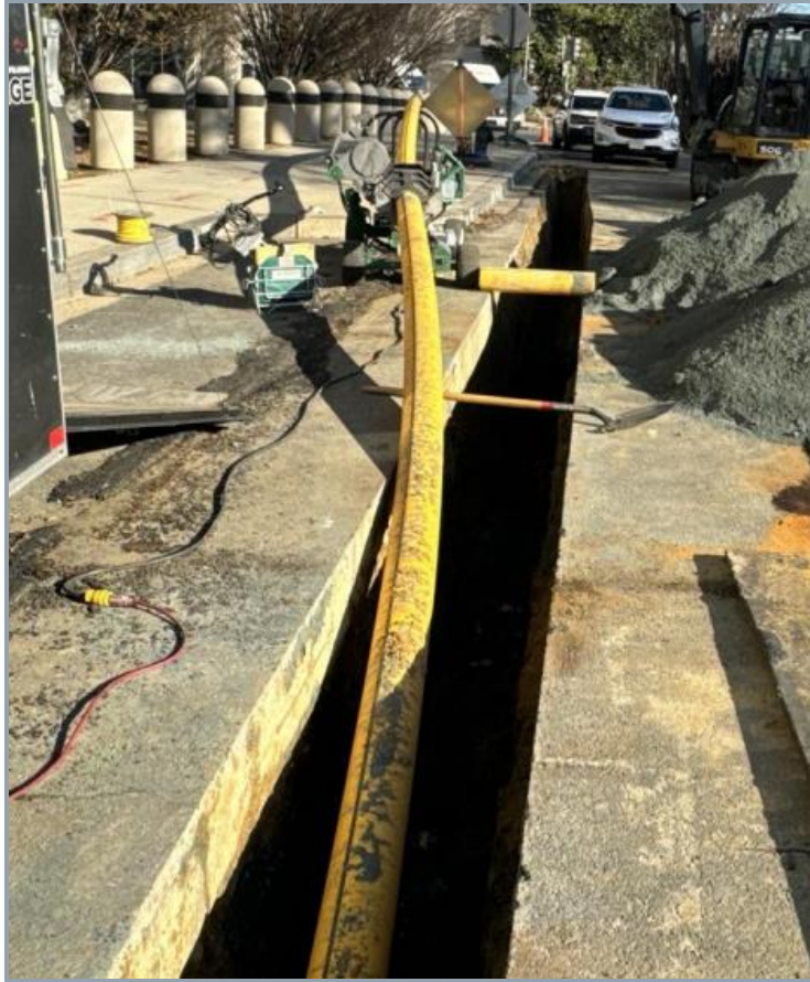
Gas line relocation
