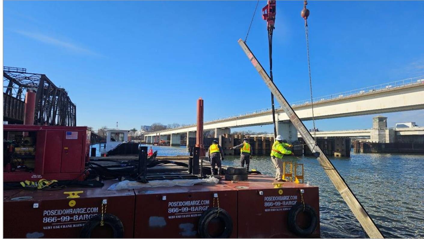
Probing underwater obstructions
