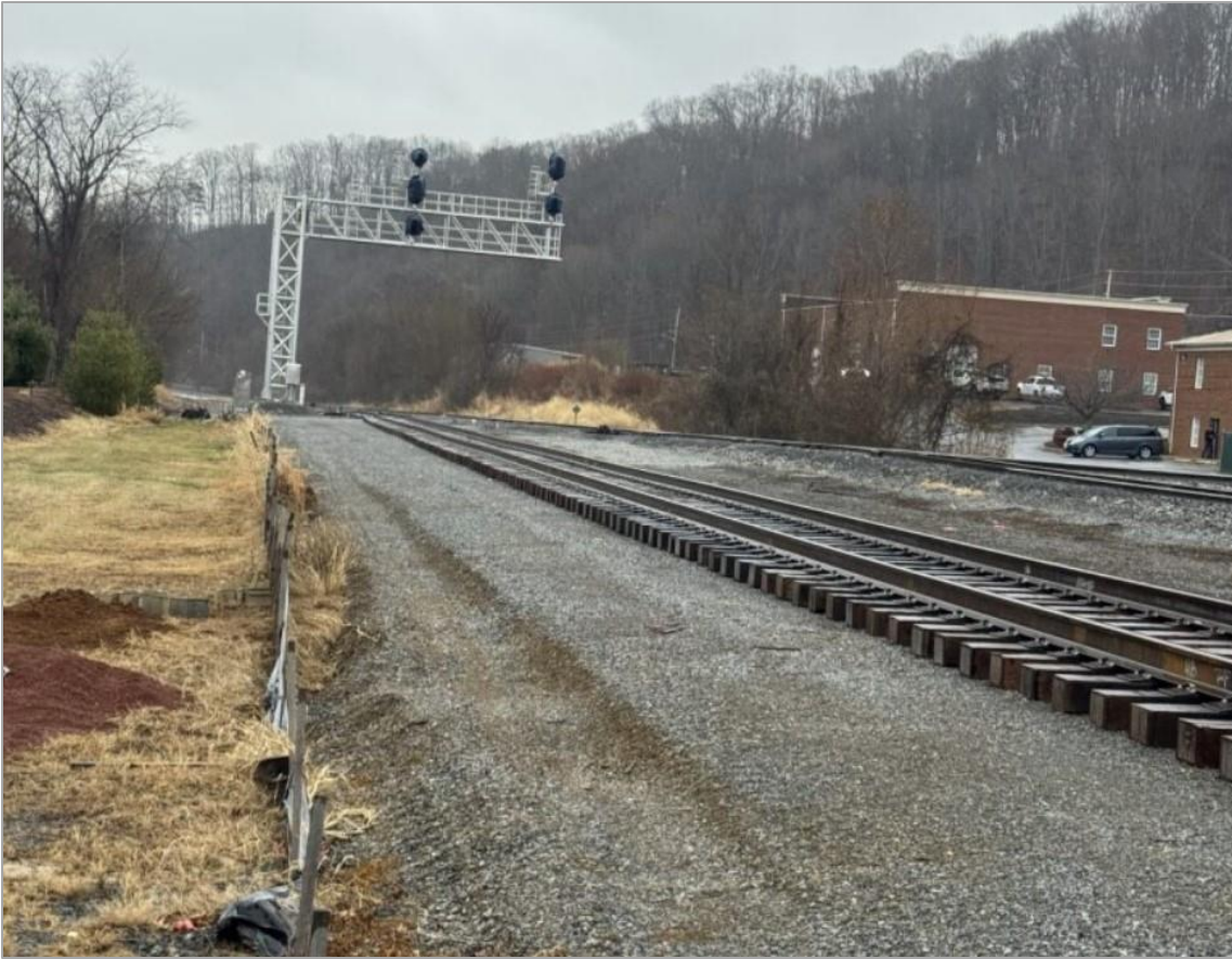
NS is installing signal infrastructure
