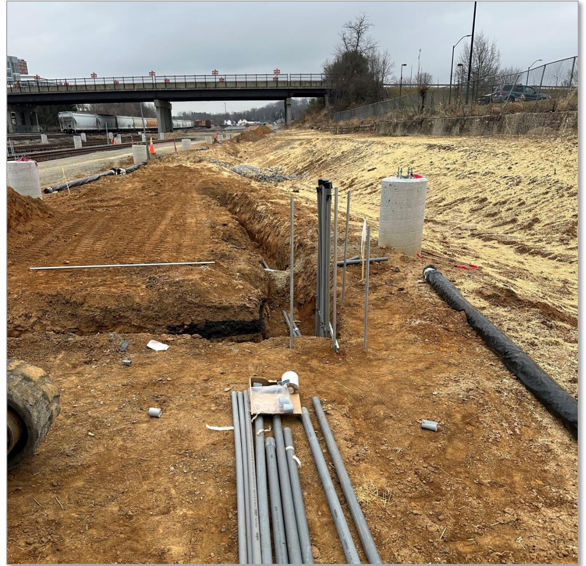
Crews are installing light poles and electrical wiring in conduits
