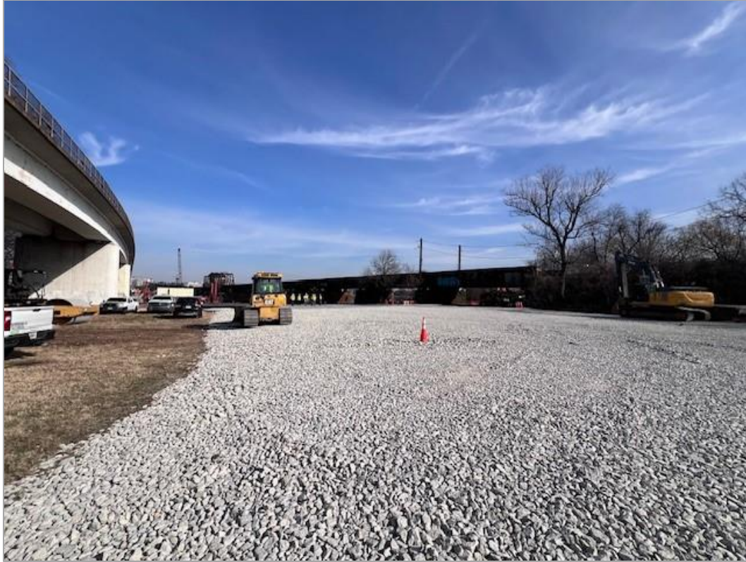
Marina Access Bulkhead preparation on Virginia shore
