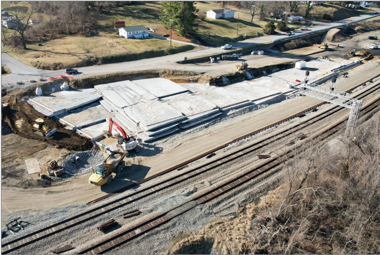
Lightweight cellular concrete placement for station parking lot
