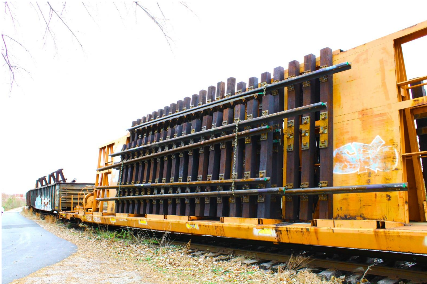
Delivery of turnout panels at Control Points AF & RO
